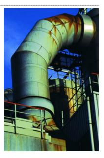
It is always wise to spend more and achieve an excellent job of surface preparation, even if the top coat selected may be compromised. A well-prepared substrate is most important because it provides a base for good adhesion of either the primer (if one is used) or the top coat. Adhesion of the coating is critical.
